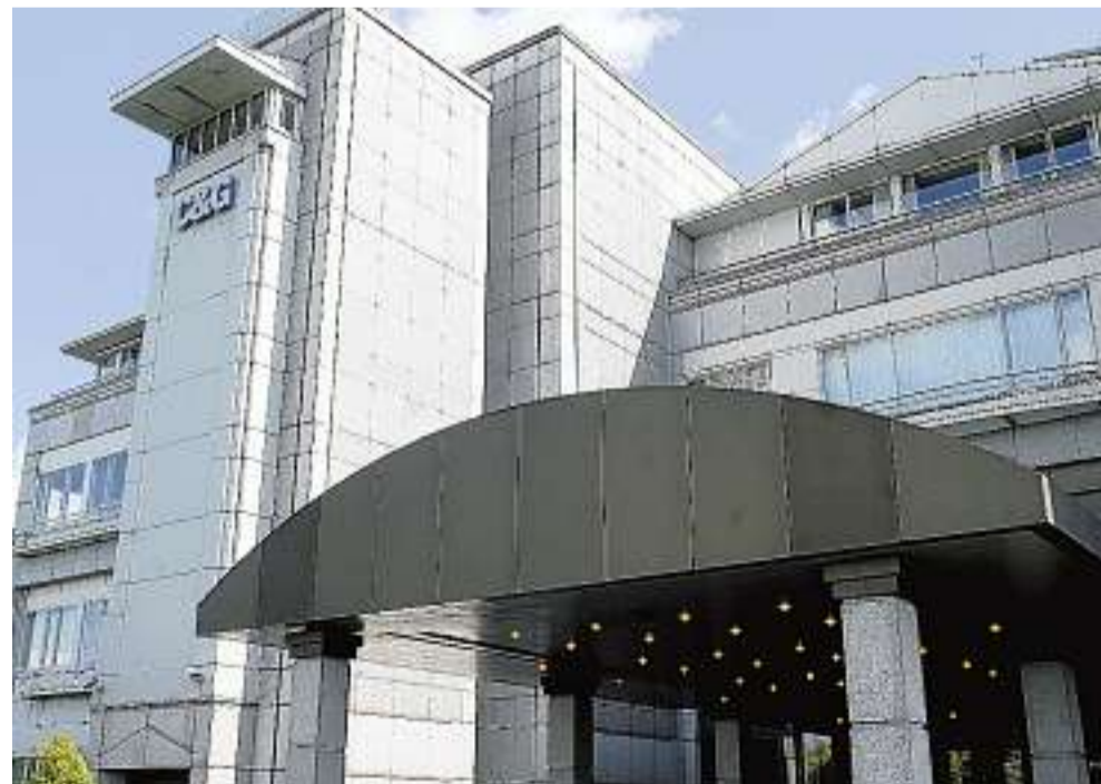
HQ: C&G offices in Barnwood
